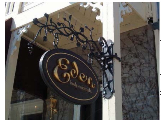
Example of custom iron work applied to façade signage armature
