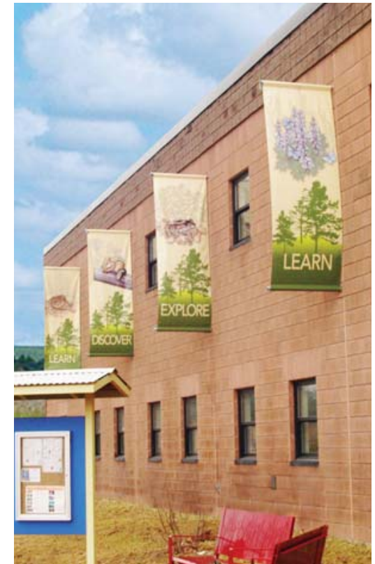
Carolinian themed public art, banners and murals should be incorporated into façades
