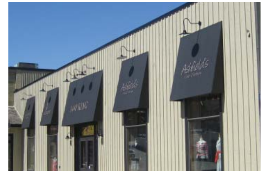
Coordinated colour palette applied to building wall and awnings strengthen the theme
